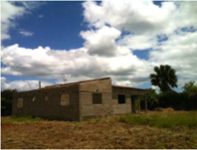
The new Manse.... and the roof goes on.
