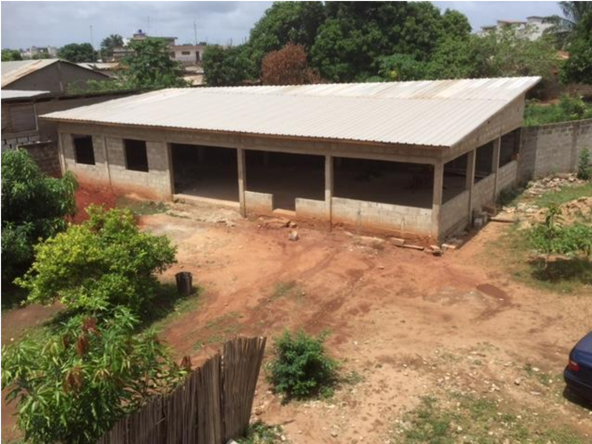
Maternity OPD under construction
